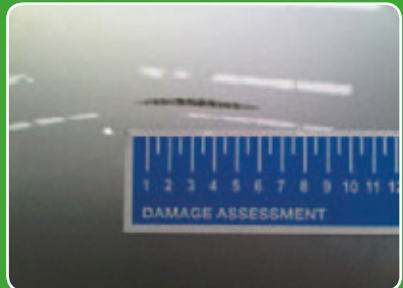
Scuff on surface not penetrating base material
